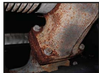
Close-up of exhaust joint
